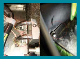
**Figure 4** (top) Gaps identified in the top of the heater-cooler water tanks **Figure 5** (right) Directional flow of air from the gaps in the top of the water tanks to the theatre environment via the fan located at the rear of the heater-cooler
